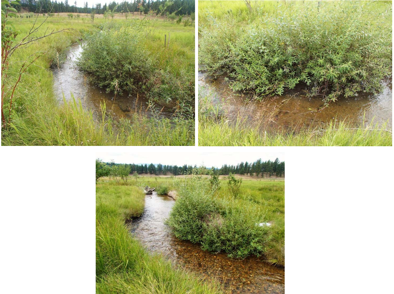
Figure 14. Photographs of willow fascines installed in Phase I. Willows in many fascines grew significantly in 2015 due to the installation of the riparian protection fence and many of these structures are providing cover and shade for the stream.
