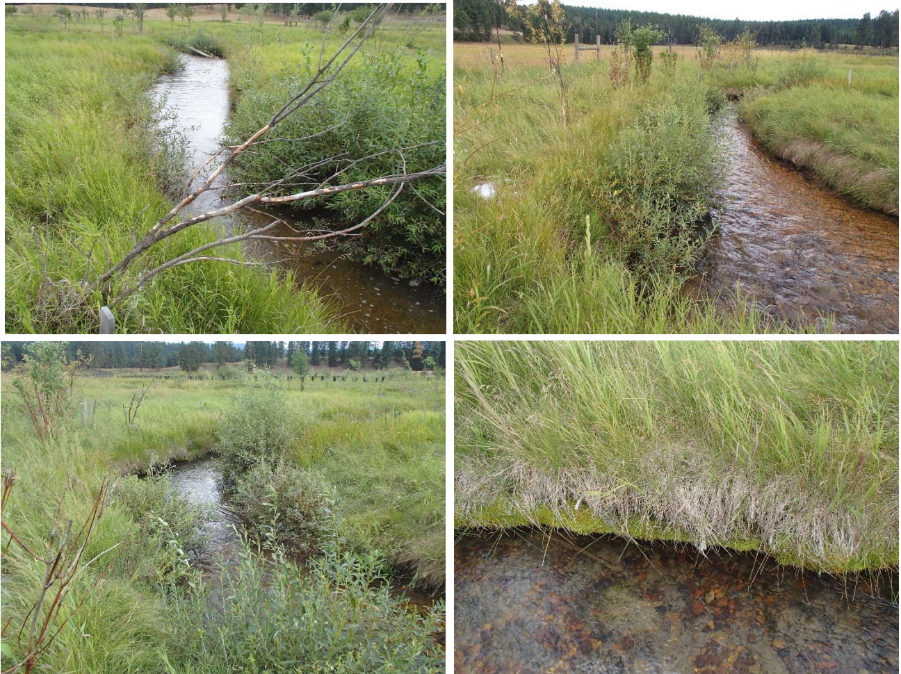
Figure 15. Photographs of coir logs installed in Phase I. In some areas, coir logs have formed dense bands of willows along the stream creating diverse habitat. In other areas, where willow survival was poor, the coir logs help support undercut banks (bottom right photograph).
