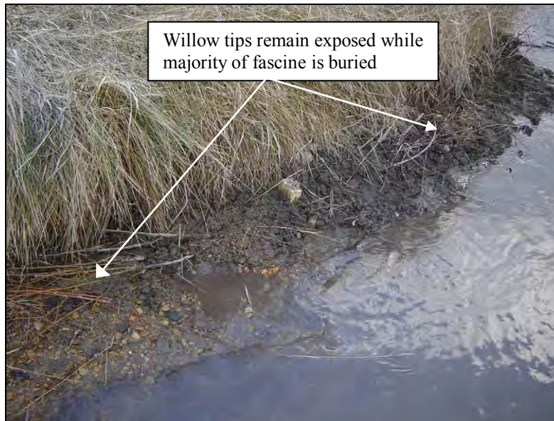
Figure A-9. Photograph of buried willow fascine treatment.
