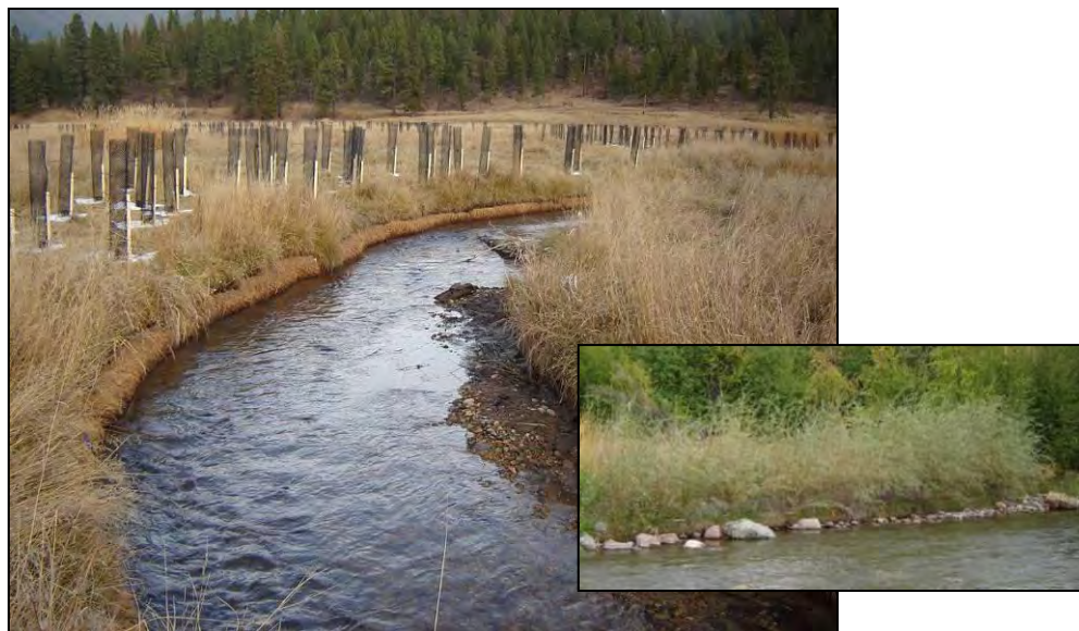
Figure A-8. Photograph of coir log immediately after installation and with willow growth after three years (inset).
