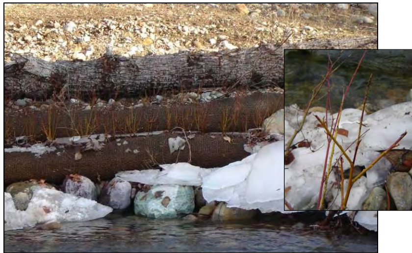
Figure 13. Photograph of vegetated soil lift bioengineered stream bank. Willows are surviving in these structures, but heavy browse (inset photo) is limiting growth and continued browse pressure could reduce survival.
