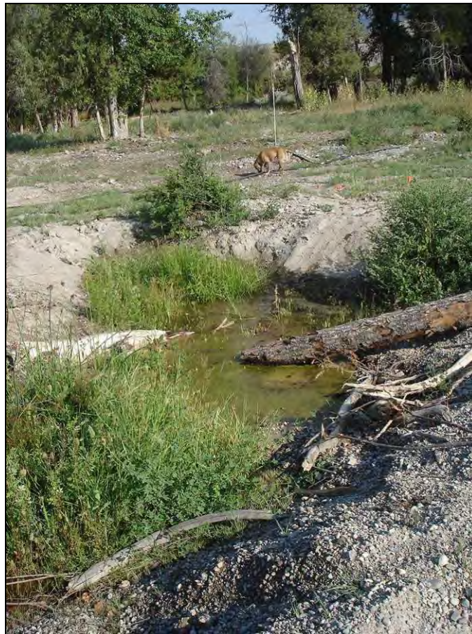
Figure A-12. Photograph of constructed floodplain swale five months after construction.
