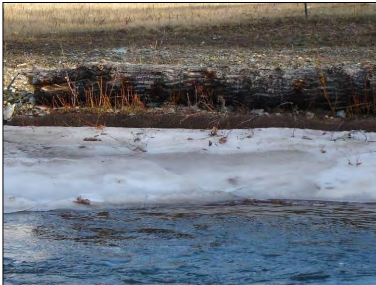
Figure 18. Photograph of soil lift 2 illustrating log barrier placed behind the structure to prevent browse. Willows are surviving but heavily browsed down to the height of the barrier.
