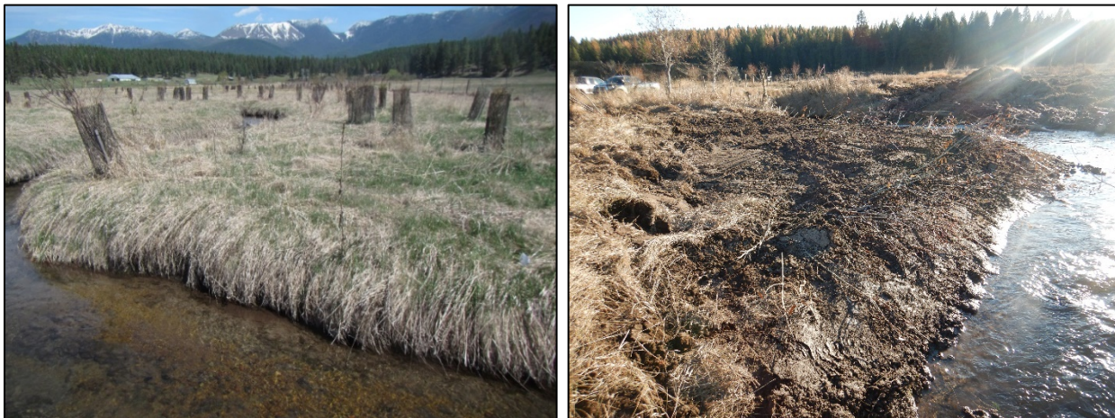
Figure 4. Point Bar Lowering Site 3 before (photo left) and after (photo right) treatment.
