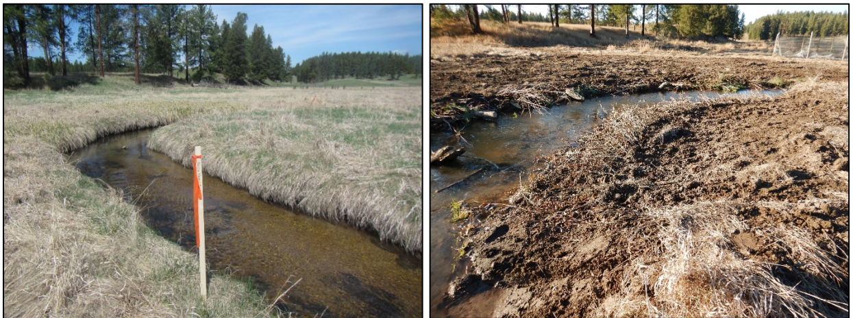
Figure 6. Point Bar Lowering Site 5 before (photo left) and after (photo right) treatment.
