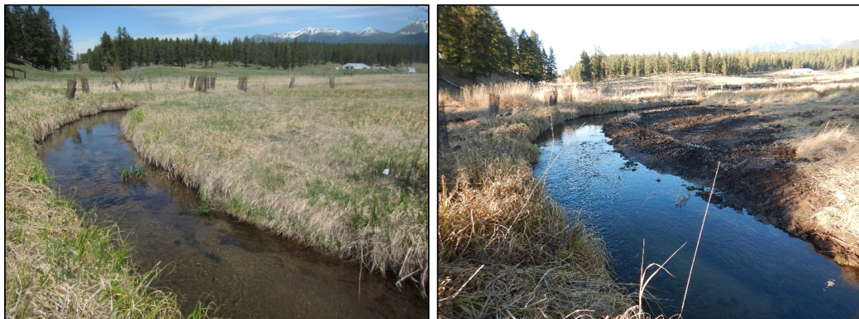
Figure 2. Point Bar Lowering Site 1 before (photo left) and after (photo right) treatment.
