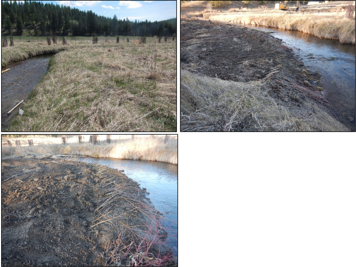
Figure 3. Point Bar Lowering Site 2 before (top left photo) and after (top right and bottom photos) treatment.
