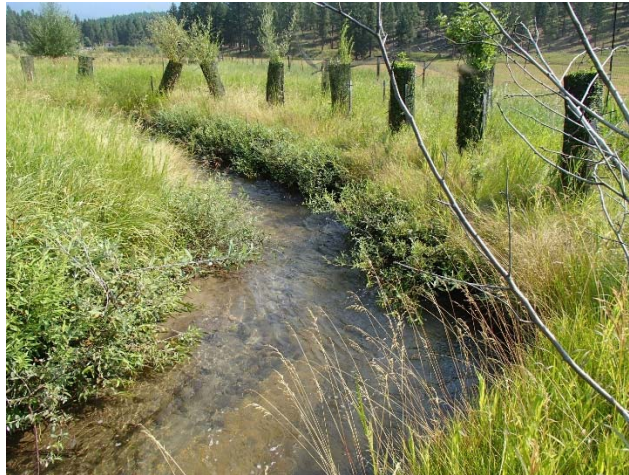
Figure 18. Coir Log 3 and willow fascine on inside bend (across from planting unit 11) showing increased height of willow cuttings.
