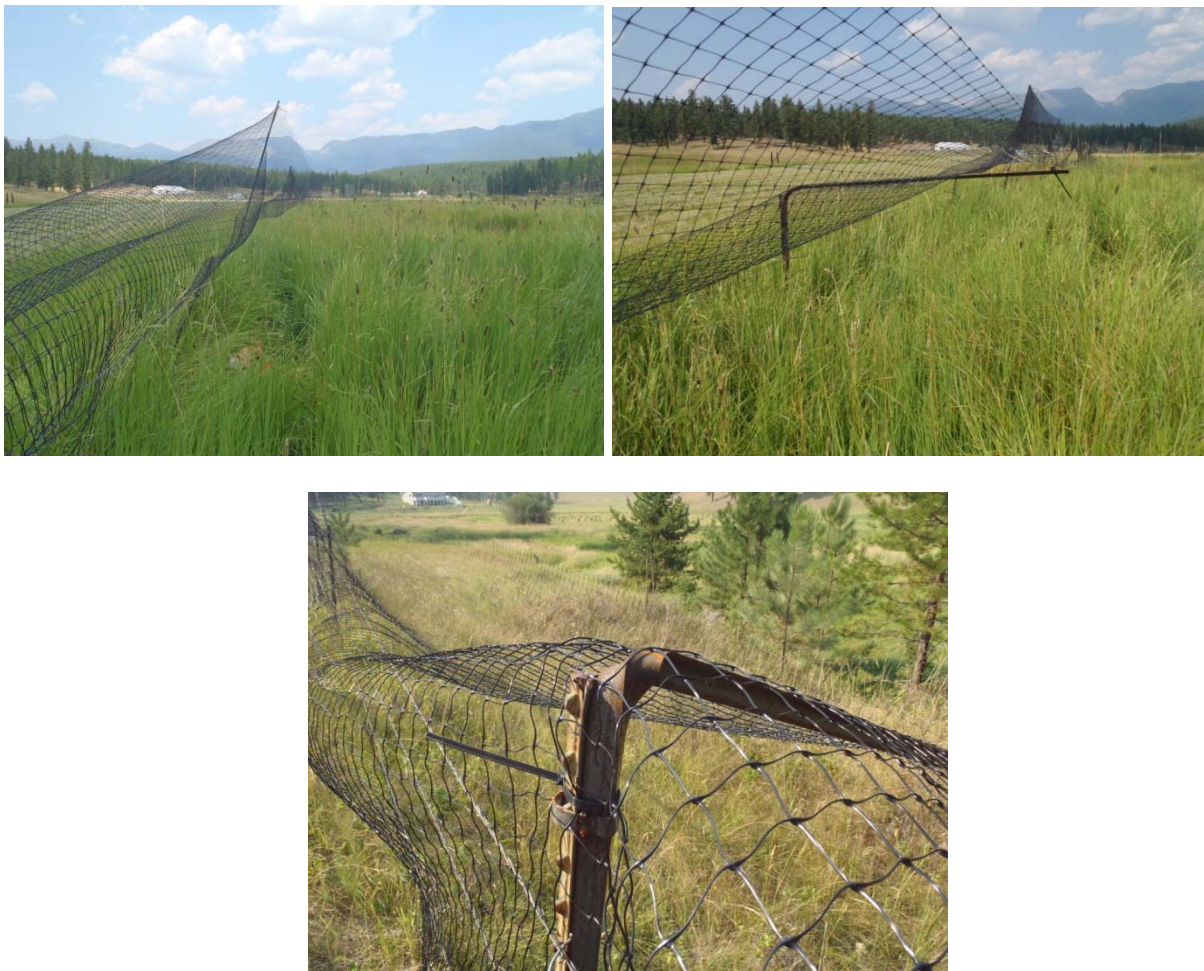
Figure 22. Photographs of riparian protection fence failure due to bending of the angle iron extensions.
