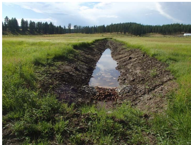
Figure 26. Drainage ditch constructed in spring 2013 in the hayfield adjacent to the project area.
