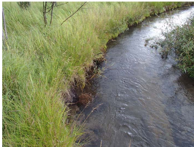
Figure 20. Coir log site where scour occurred at the upstream end of the structure during 2012 high flows. Bank erosion resulted in a vertical bank upstream of the coir log but the vegetated under-cut bank was maintained where coir logs were left intact.
